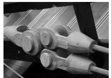
Anchoring of Capilano Bridge
