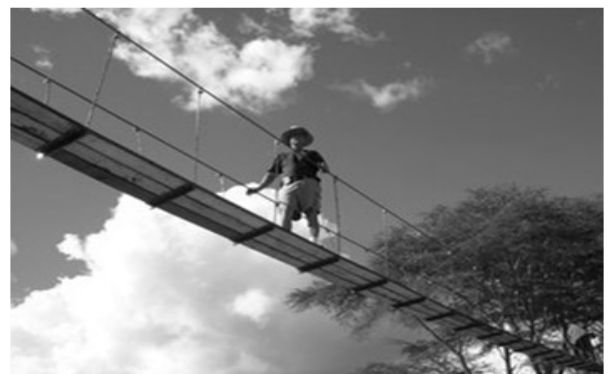
One of Harmon's bridges
