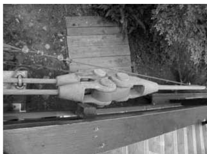
Anchoring of Capilano Bridge
